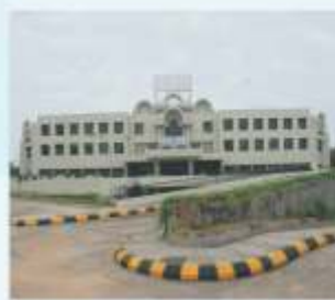
METRO HOSPITAL & RESEARCH INSTITUTE, Vadodra
